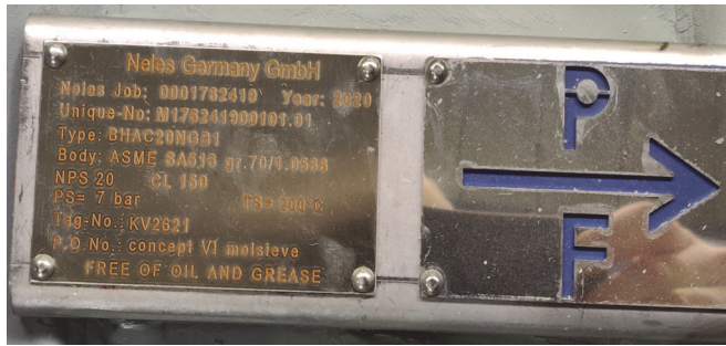
Fig. 3 Example of id-plate and pressure/flow direction
